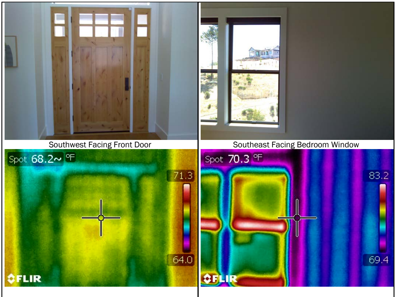
Figure 19: Standard and Thermal Photos of Region A Home (New Construction Interior)
