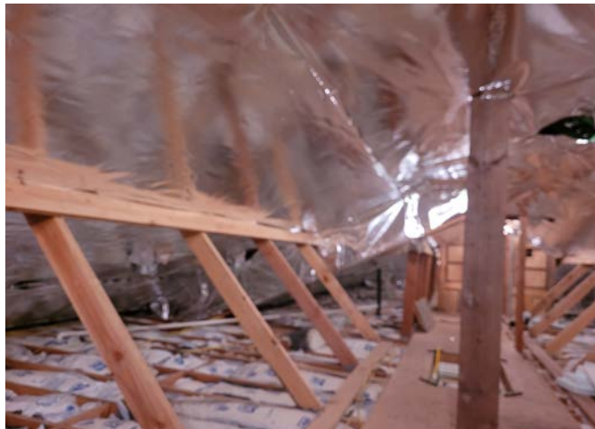
Figure 16: Attic with Insulation and Radiant Barrier (Non-perforated)
