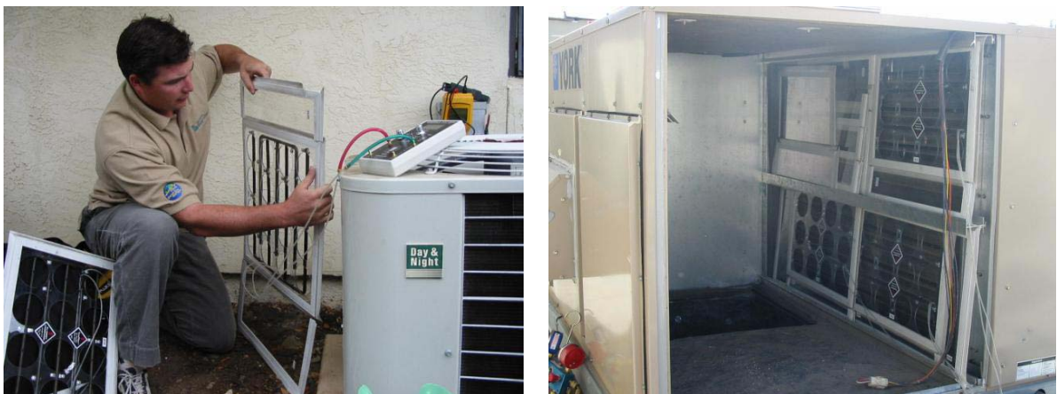
Figure 7.10: Airflow Measurements Using a Flow Grid
