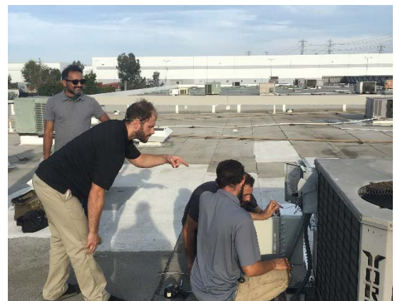
Figure 2-2. Commercial packaged RTU
