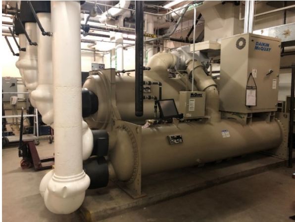
Figure 2-5. Water-cooled chiller
