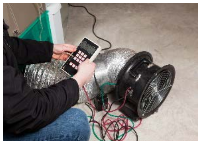
Figure 2-4. Residential air duct testing prior to sealing
