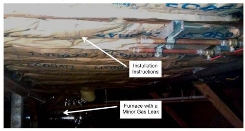
A minor gas leak was detected at the furnace using the gas leak detector. A soap bubble solution indicated a very slow bubble. There was a developing bubble and it was steady.
