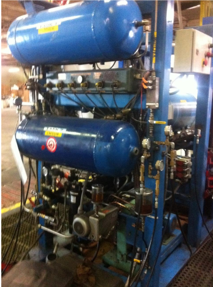
Figure I-8. Refrigerant Removal Equipment (JACO Fullerton Facility)
