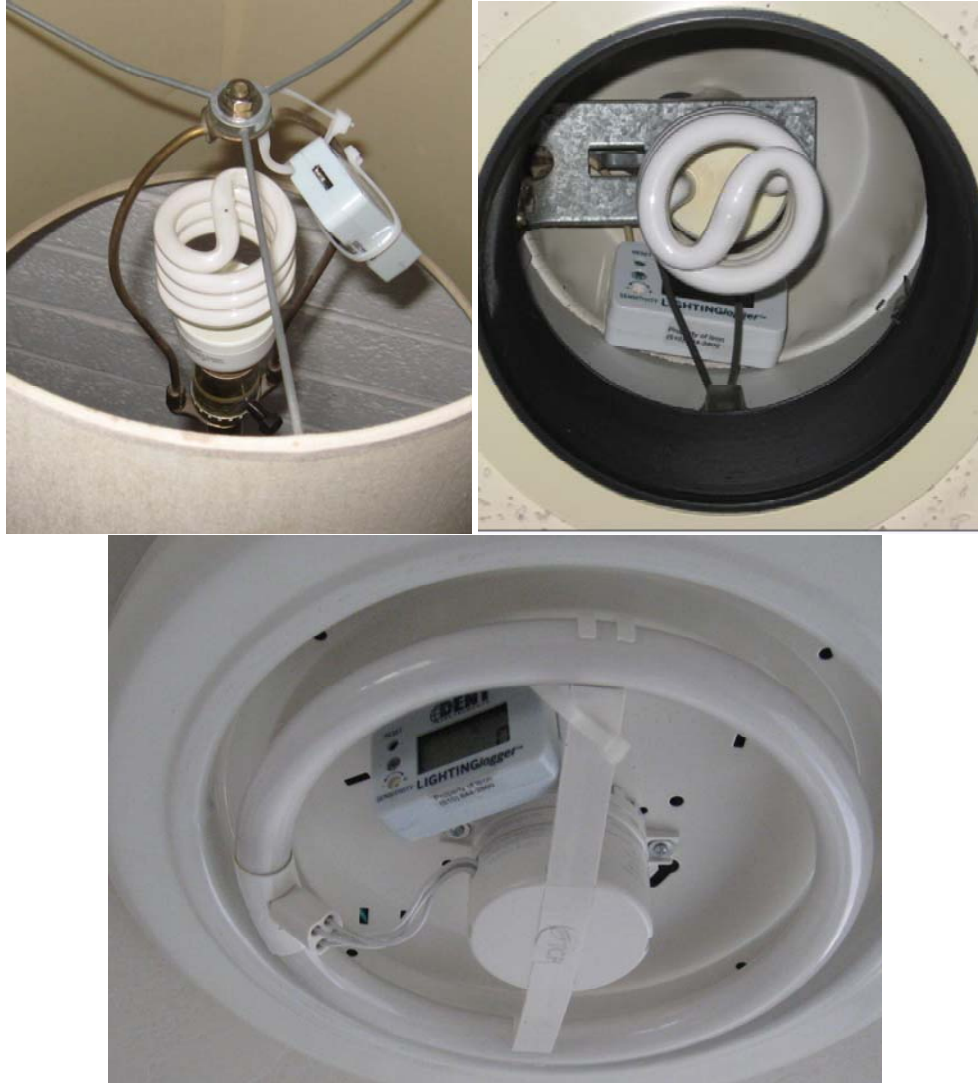
Figure J-1: Photos of Logger Installations
