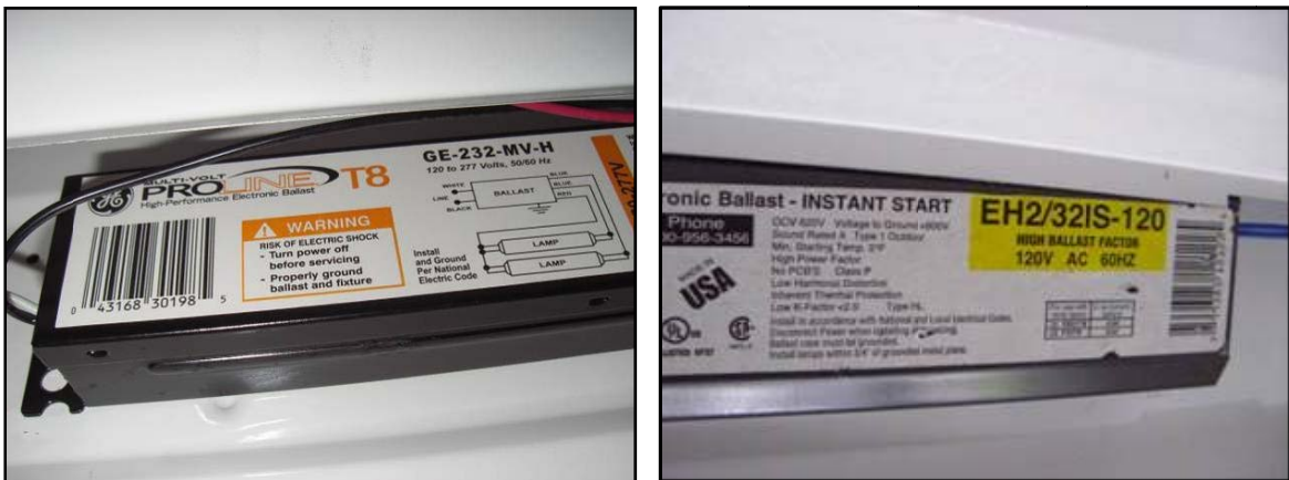
Figure B-18 Ballast Label Photos Showing Make and Model Numbers
