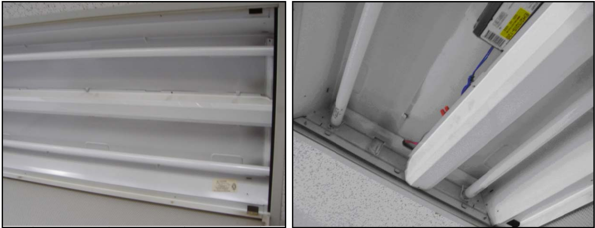
Figure B-16: Ballast Cover in Place and Unlatched/Revealed
