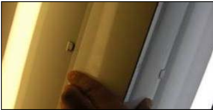
Figure B-17: Ballast Cover Clips
