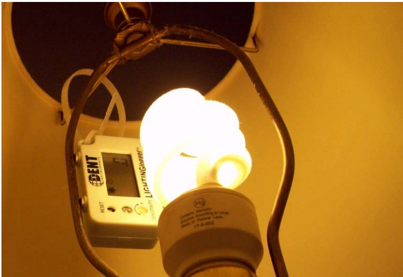
Figure B-5: LL Logger Installation in a Table Lamp w/ Zip Ties
