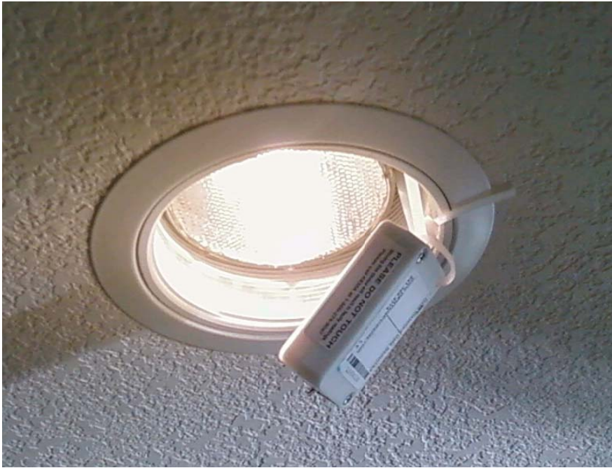
Figure B-4: LL Logger Installation in a Downlight w/ Zip ties
