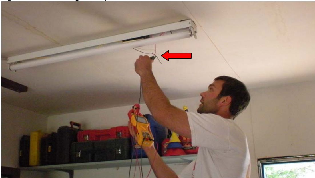
Figure 5. Connect Alligator Clip From Common Terminal to Neutral Wire
