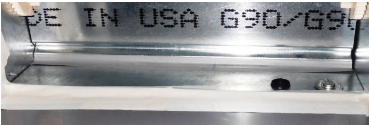
Figure 36: Sealed Economizer for 3-ton non-TXV RTU5 with Tape around Perimeter
