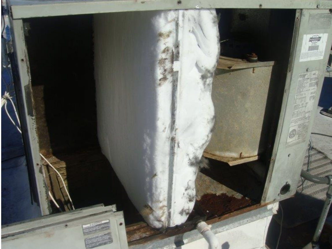
Figure 13: Dirty Frozen Air Filter and Evaporator Coil Caused by Excessive Blockage
