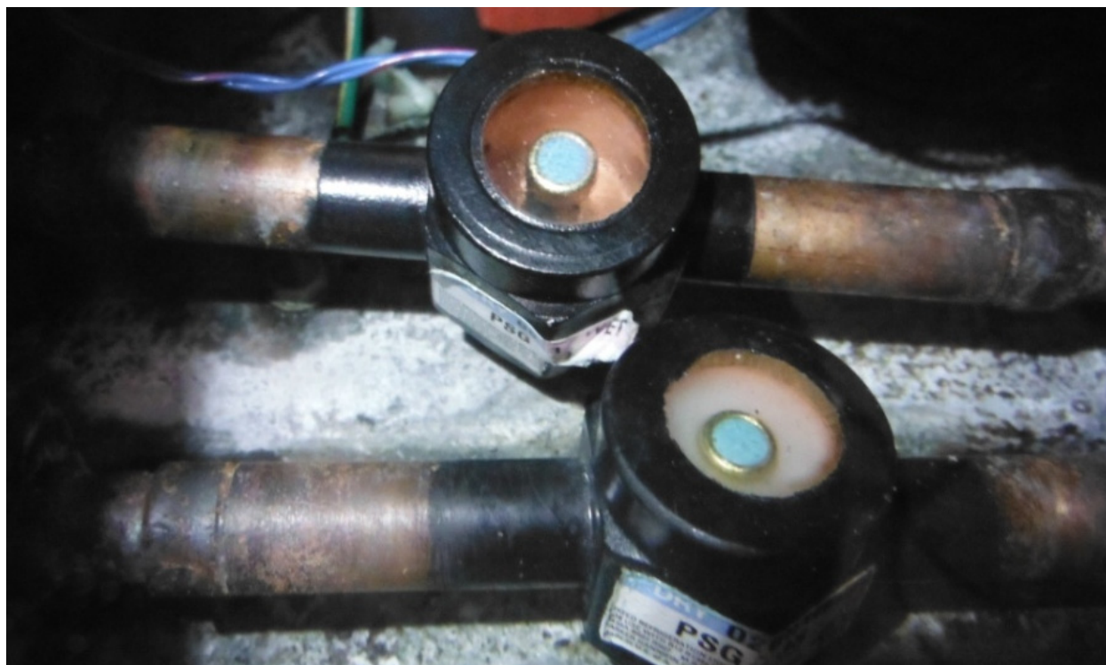
Figure 28: Sight Glass FDD Shows White Bubbles in C1 with 90% Factory Charge
