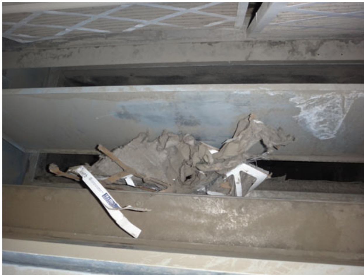
Figure 16: Evaporator Blockage with Dirty Filter Blocking Economizer Return Damper
