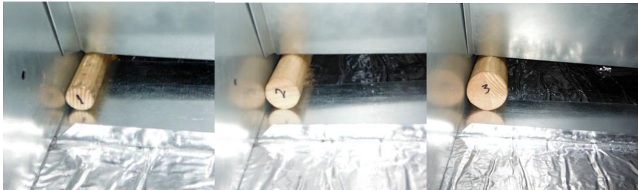
Figure 3: Economizer #1 Damper Positions Using 1, 2, and 3-Finger Dowels
