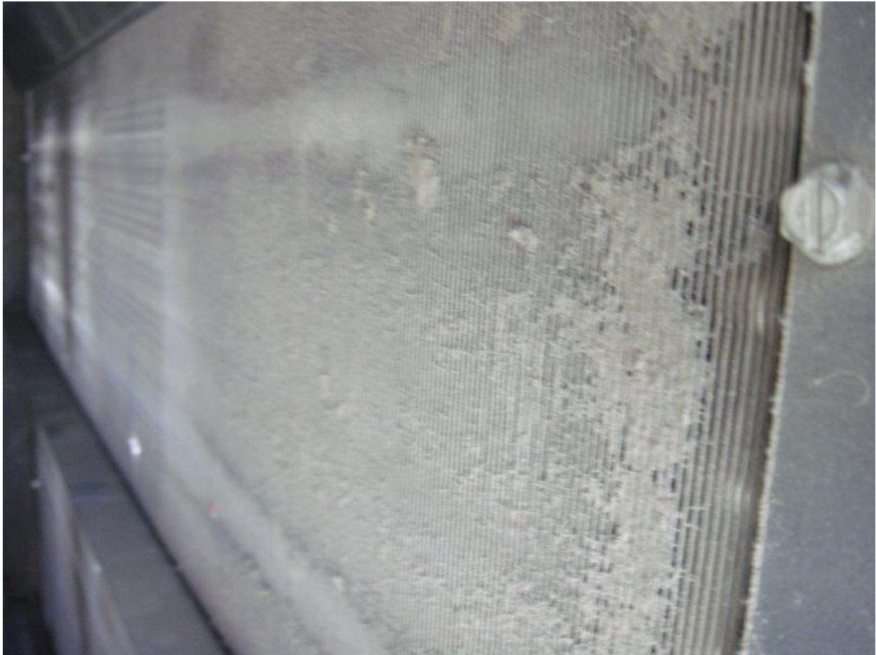
Figure 15: Evaporator Coil Blockage with Dirt Blocking 50% of the Coil
