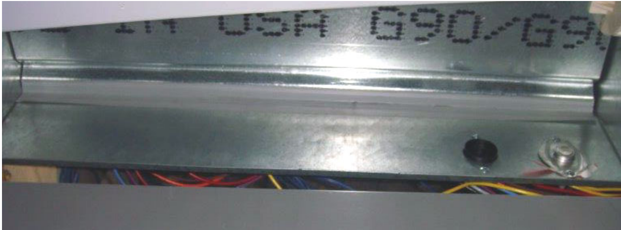
Figure 35: Unsealed Economizer Perimeter for 3-ton non-TXV RTU5 (wires showing through gap)
