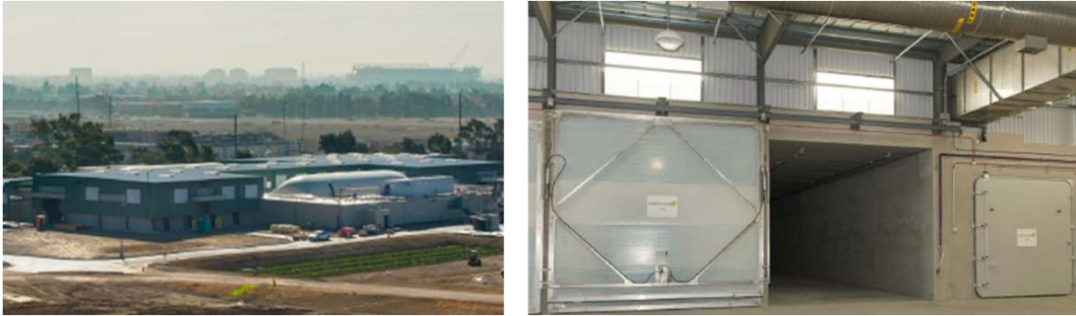
Figure 21: Zero Waste Site (Left) and Dry Fermentation Cells (Right) (Courtesy Zero Waste)
