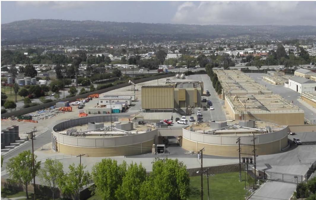
Figure 19: Los Angeles County Sanitation District (Courtsey LACSD )
