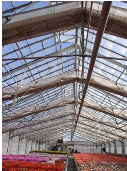
Photograph 1: Furled Greenhouse Heat Curtain
