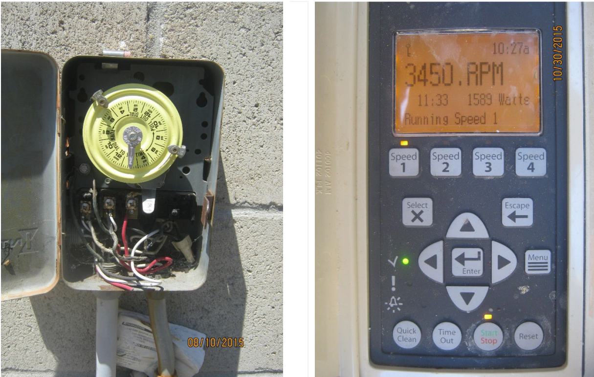
Figure 3-2 Typical Dial Timer used to Control Pool Pumps (left) and a Variable Speed Pump Control Panel (right)
