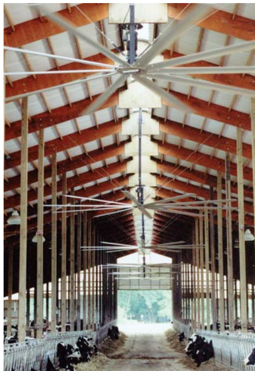
Figure B–2. HVLS Fans in Dairy Barn
