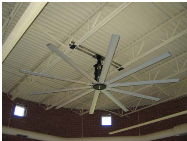
Figure B–1. HVLS Fan
