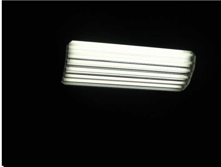
Figure 3–2. High Bay Six-Lamp High Light Output T-8 Fixture 304
