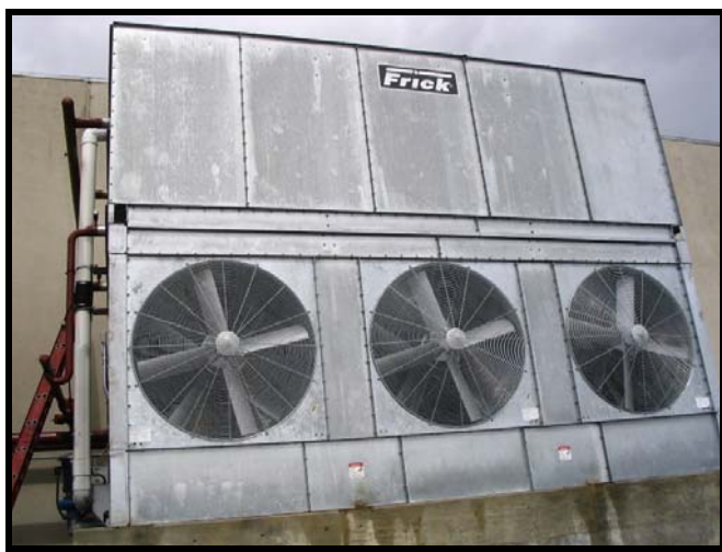
Figure 3–6. New Imeco (Frick) XL 785 Evaporative Condenser 313
