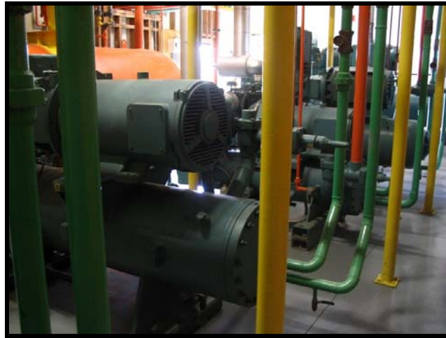
Figure 3–5. Compressors (New Frick RWF 177 at End) 312
