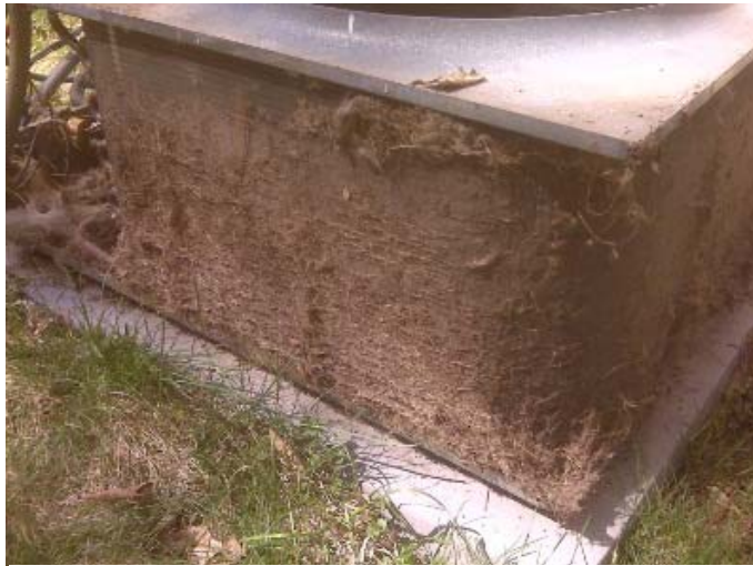
Figure 3. Condenser Coil Fouling
