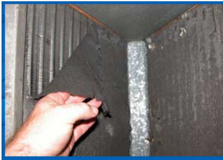
Figure 4. Evaporator Coil Fouling
