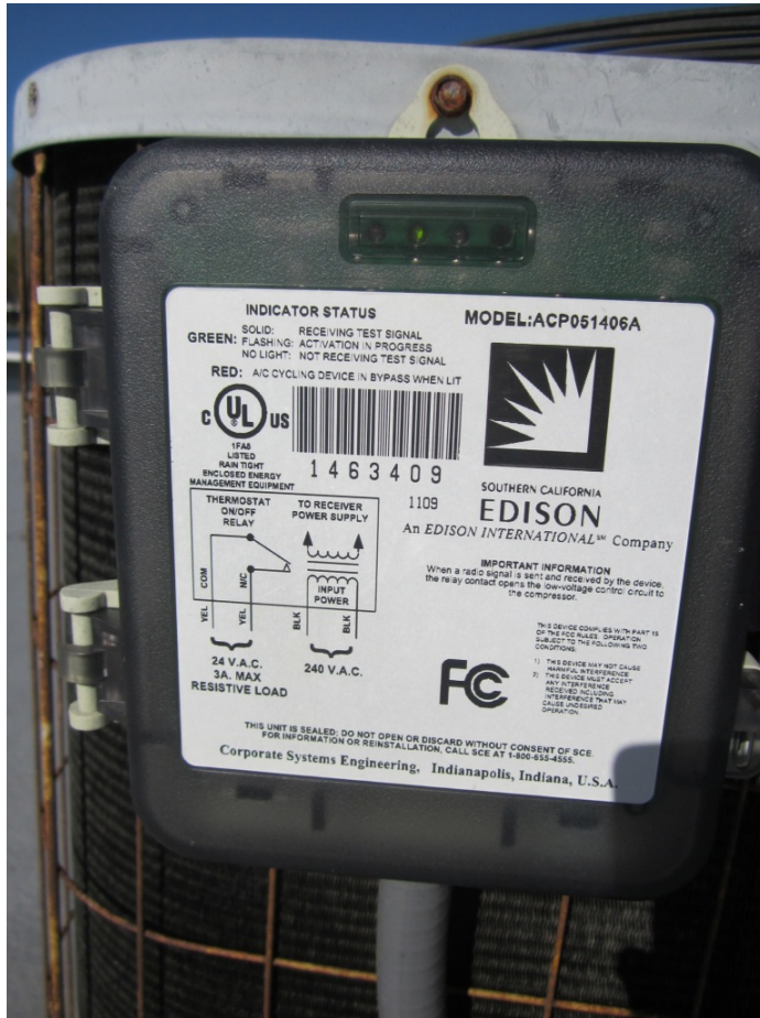
Figure 5-12: Example of Utility-Controlled A/C Demand Response Unit
