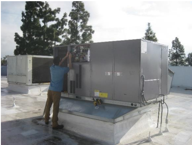
Figure 2-3. Packaged commercial rooftop unit (RTU)
