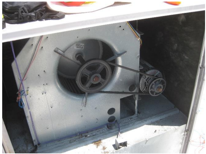
Figure 2-4. Supply fan in RTU
