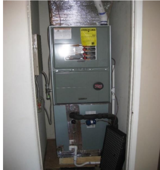
Figure 2-2. A typical high-efficiency residential furnace
