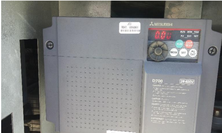
Figure 2-7. Fan motor VFD control inside an RTU
