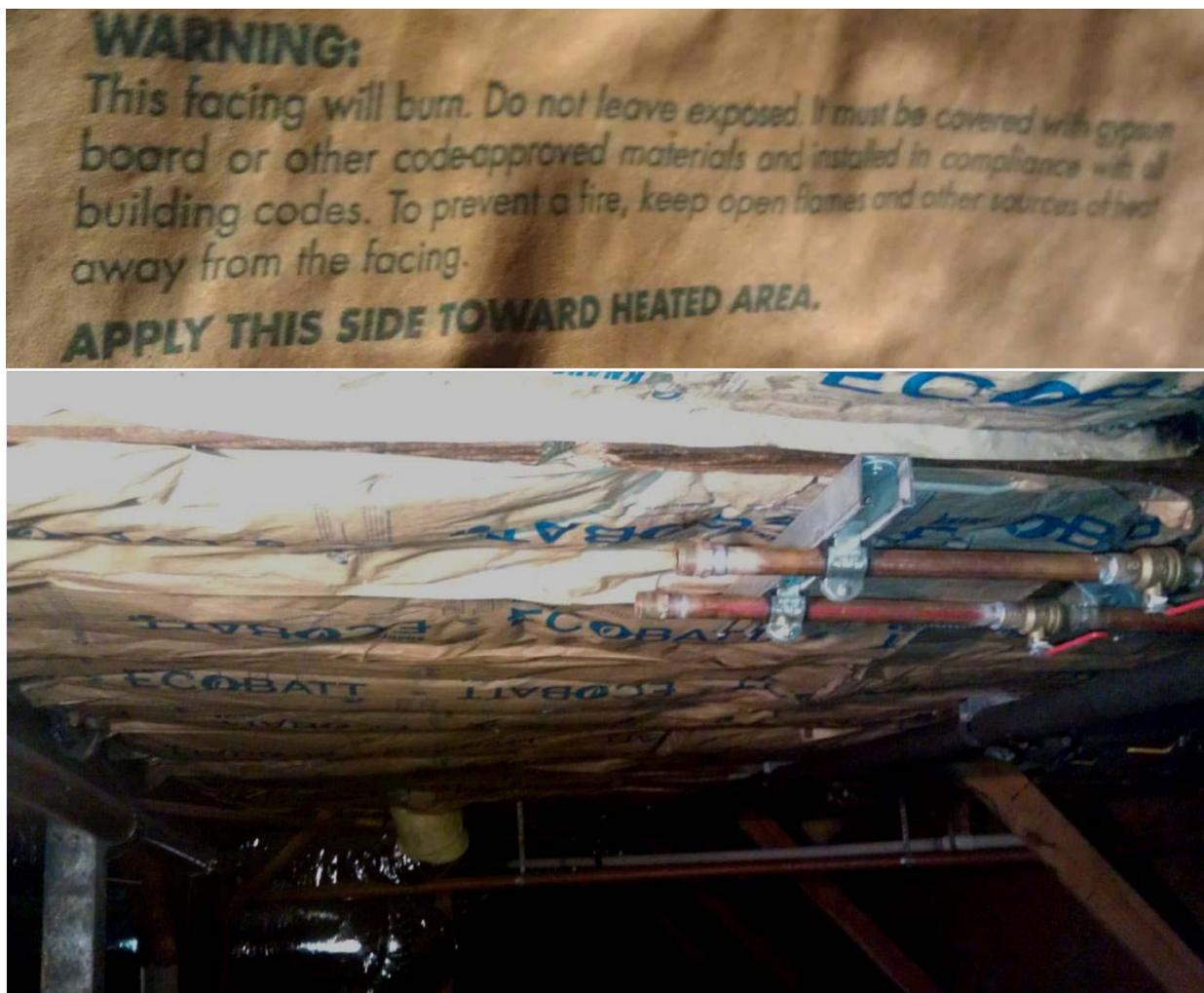
**Figure 14: Apparent Instance of Fire and Mold Hazard**
