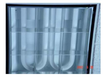
Figure 8. Typical 2 foot by 2 foot T-12 U-Tube fixture
