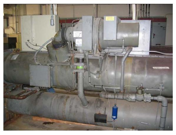
Figure 14. Existing 120-Ton Screw Chiller
