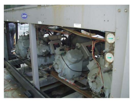
Figure 11. Completed Turbocor Chiller Retrofit
