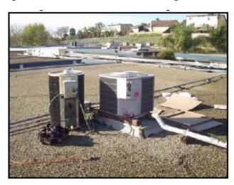
Figure 9. Old and New Units During Installation
